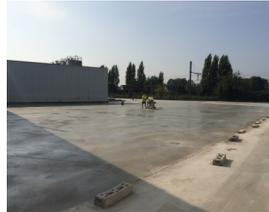
**Applying saw cuts within 24 hours**
