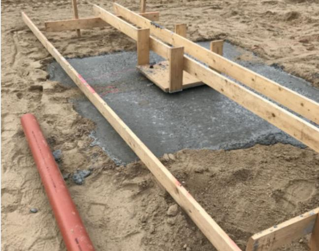
With Durus S500 fibres already contained in the concrete when it is delivered to site, many point foundations can be poured in one time, which greatly reduces construction time.
