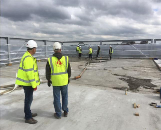
The use of DURUS S400 allows large areas to be flood poured without any risk of disturbing in-situ steel mesh reinforcement. Insufficient concrete cover is also not a factor as the reinforcement comes ready mixed in the concrete, which can be easily pumped into position.
