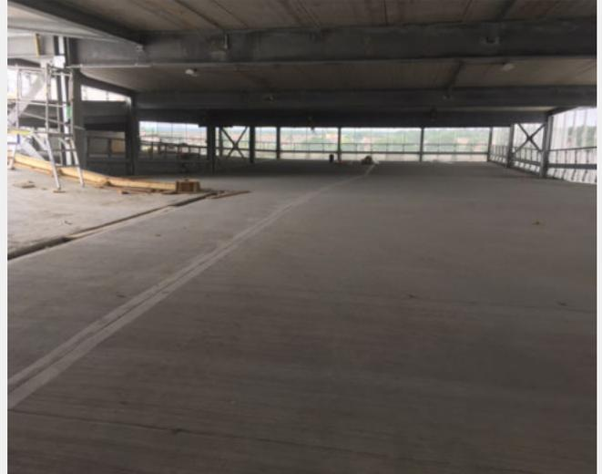
Owing to the confined working area, the handling cutting and fixing of steel mesh would present significant health & safety hazards during installation of the topping, and would also be very time consuming.
