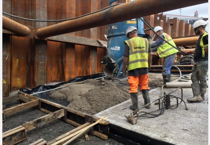
The confined nature of the site would make it difficult and dangerous to handle, cut and fix welded steel fabric. The DURUS S400 Macro Synthetic Fibre Reinforcement is contained within the concrete on delivery, so cannot be placed incorrectly or disturbed during installation.
