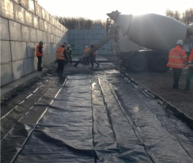
With the **DURUS S400** Synthetic Macro Fibre reinforcement already contained in the concrete when it is delivered to site, large areas can be poured which greatly reduces construction. Saw cut contraction joints can then be cut 1/3 of slab depth, within 24hrs of placement and finishing.
