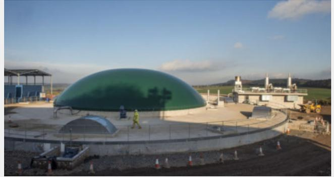
One of the 48m diameter Tanks in which the silage is broken down to produce gas fuel which is burnt to heat water. The resulting steam powers turbines to make electricity.
