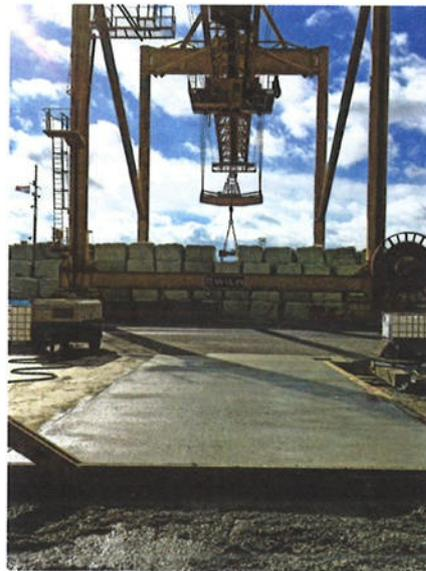
Above: Installation and finishing of macro-synthetic-fibre-reinforced concrete at the Port of Tyne.
