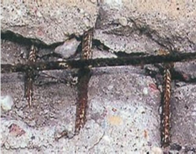
The use of welded steel mesh reinforcement would lead to a shortened service life due to corrosion in this marine environment.
