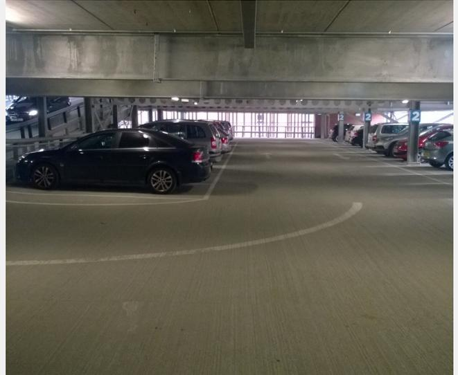
A brush finish was given to the Screed Topping. The Client was very happy with the aesthetics and consistency of the finished surface.
