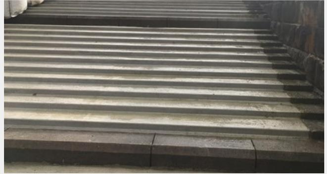
Some of the original Stone Masonry is reused with the remaining concrete channels installed with a Fibre Mix.
