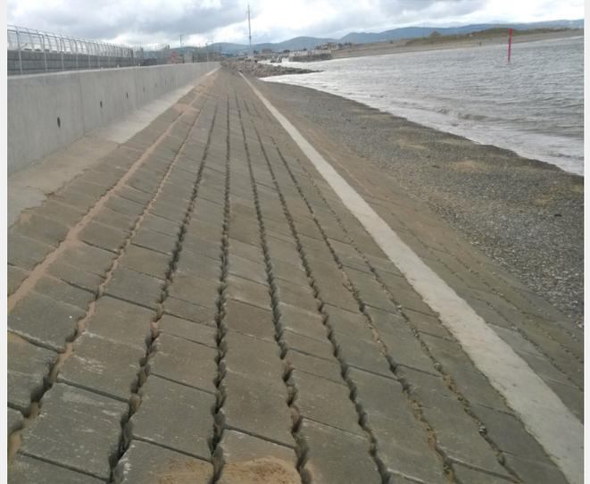
Linked Concrete blocking surrounded by C40 Concrete containing 4Kg Durus S400. Protecting the Land from coastal attack & Erosion
