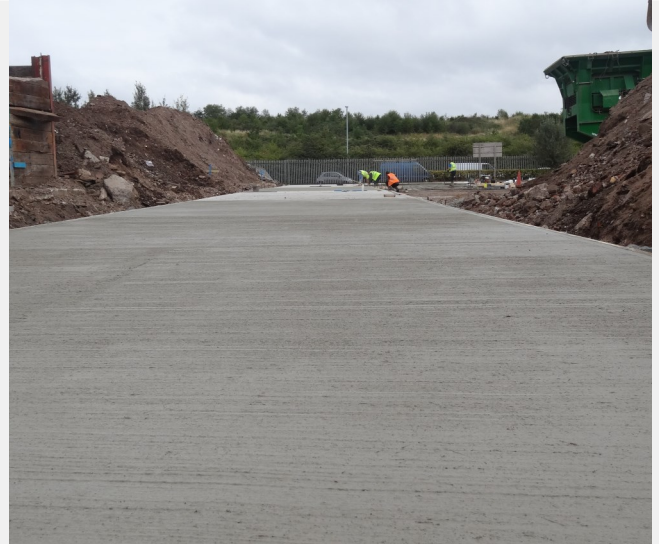
Brushed finish with saw cuts at 6 meter spacing's
