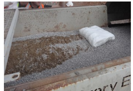
Durus S400 going on with the sand and aggregates. 1 Bag every 30 seconds
