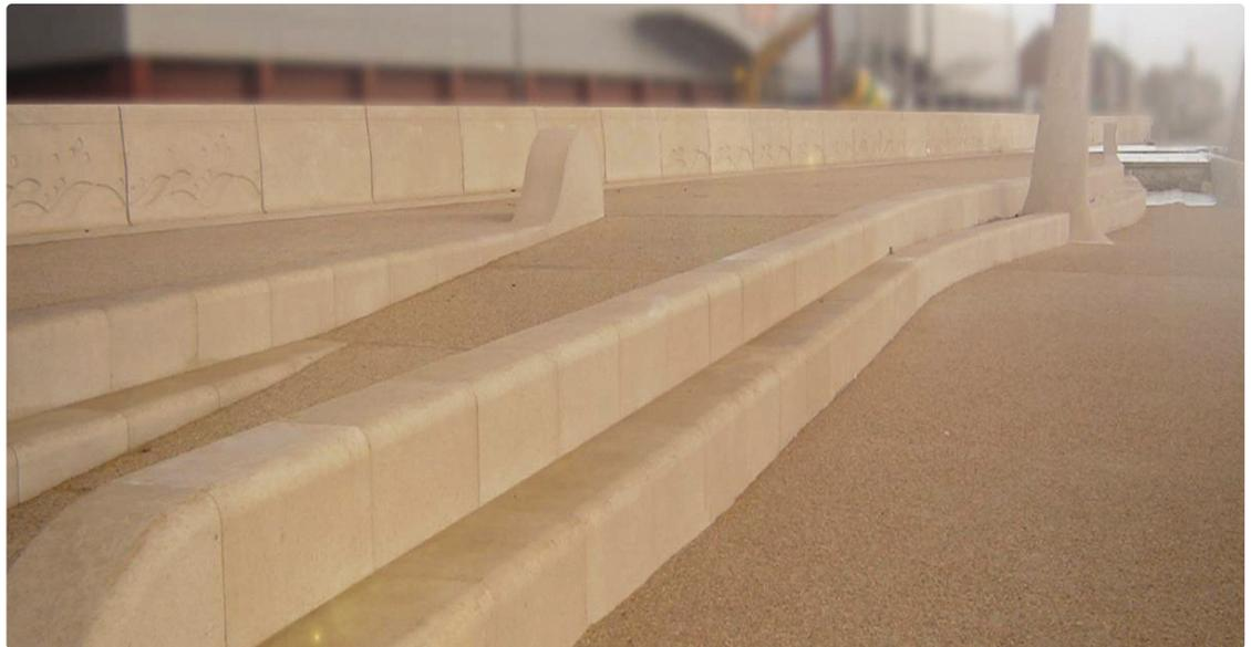
**Figure 4 right: Ovingdean and Brighton Marina sea wall and ramp containing Fibrin Fibres.**
