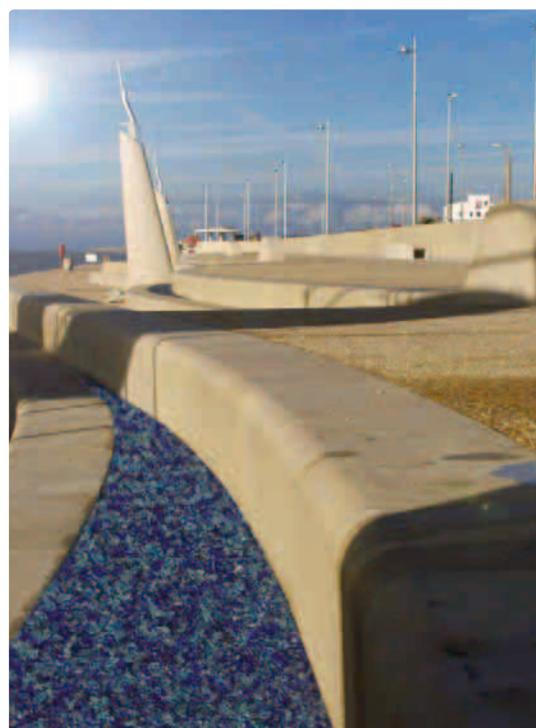
**Figure 2: Cleveleys promenade containing Fibrin XT polypropylene fibres.**
