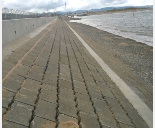
Linked concrete blocking surrounded by C40 concrete containing 4 kg Durus S400. Protecting the land from coastal attack and erosion.
