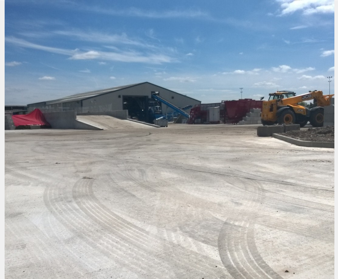
The addition of Fibrin XT gives enhanced abrasion and durability, important in this application, due to tyre scrub from turning vehicles
