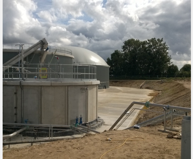
Macro fibre reinforced concrete eliminates the use of steel and the risk of shortened service life due to corrosion and spalling.
