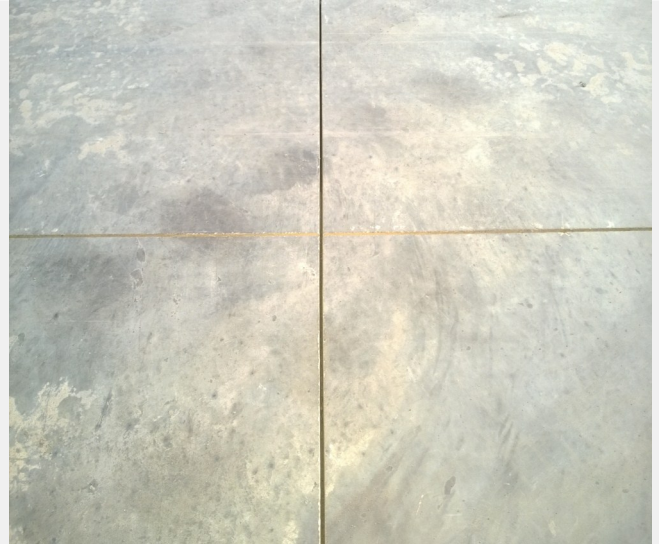
Power floated finish with saw cuts at 6 meter spacings
