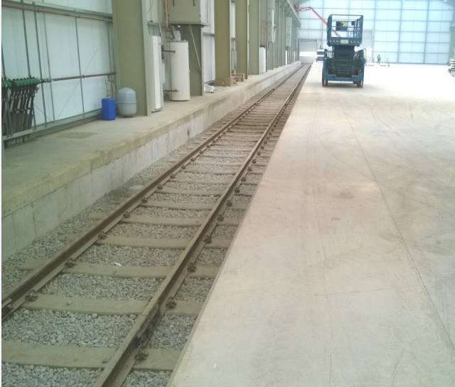
Rail line inside the building
